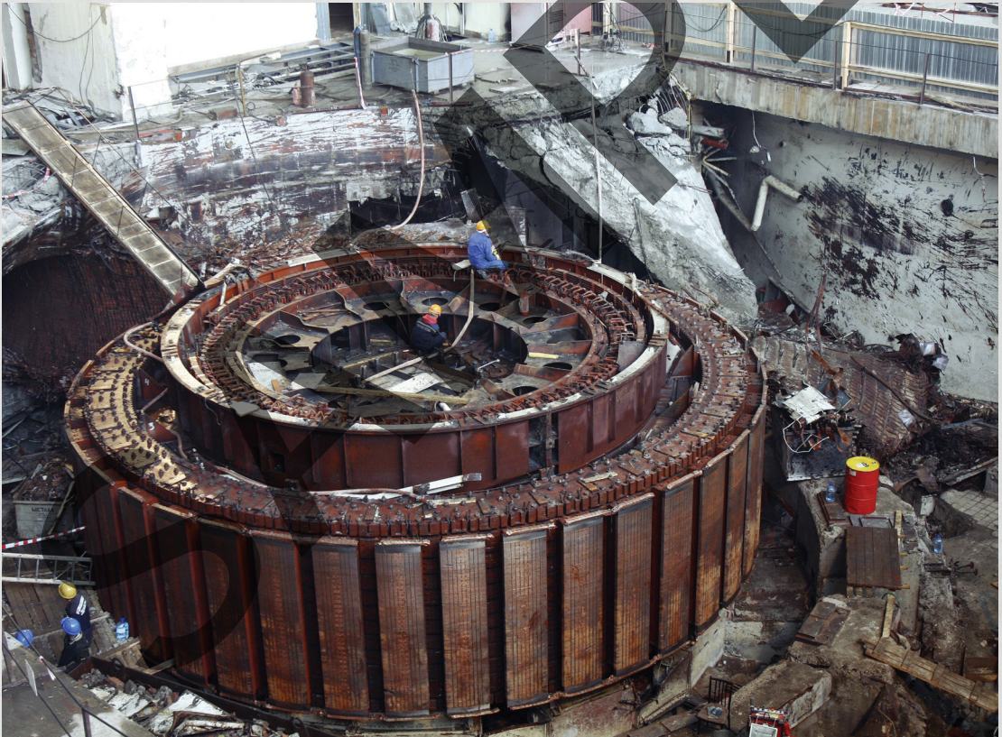
Workers cleaned up after the accident.
