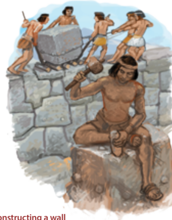
Constructing a wall
